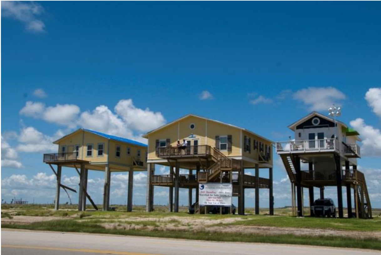
FIGURE 1.1: Gilchrist, Texas, Aug. 16, 2009. These stilt homes were the only structures still standing in the town of Gilchrist after Hurricane Ike destroyed it. FEMA is still working with local, state, and federal agencies to rebuild the town. Photo by Patsy Lynch/FEMA.
