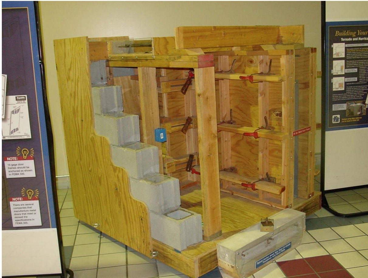
FIGURE 2.6: Tulsa, Oklahoma, Nov. 23, 2001. Disaster Ally in the Eastland Mall. Safe rooms can be designed with many different materials. Shown are concrete block walls, formed concrete walls, and a special ceiling framing. Photo by Kent Baxter/FEMA News Photo.
