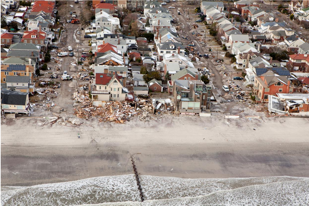
FIGURE 2.1: Long Beach, N.Y., Nov. 8, 2012—Aerial views of Hurricane Sandy damage to homes on Long Beach, New York. Following the hurricane, a nor'easter struck the area causing more power outages and additional flooding. FEMA is working with state and local officials to assist residents who were affected by Hurricane Sandy. Andrea Booher/FEMA.
