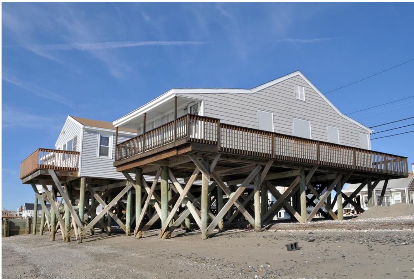
FIGURE 3.1: Stratford, Connecticut. December 6, 2012—These summer cottages are examples of homes not severely damaged by Hurricane Sandy due in large part to being elevated on pilings. FEMA is in the area with mitigation specialists who are knowledgeable about the value of pilings to support coastal homes. Photo by Marilee Caliendo/FEMA.
