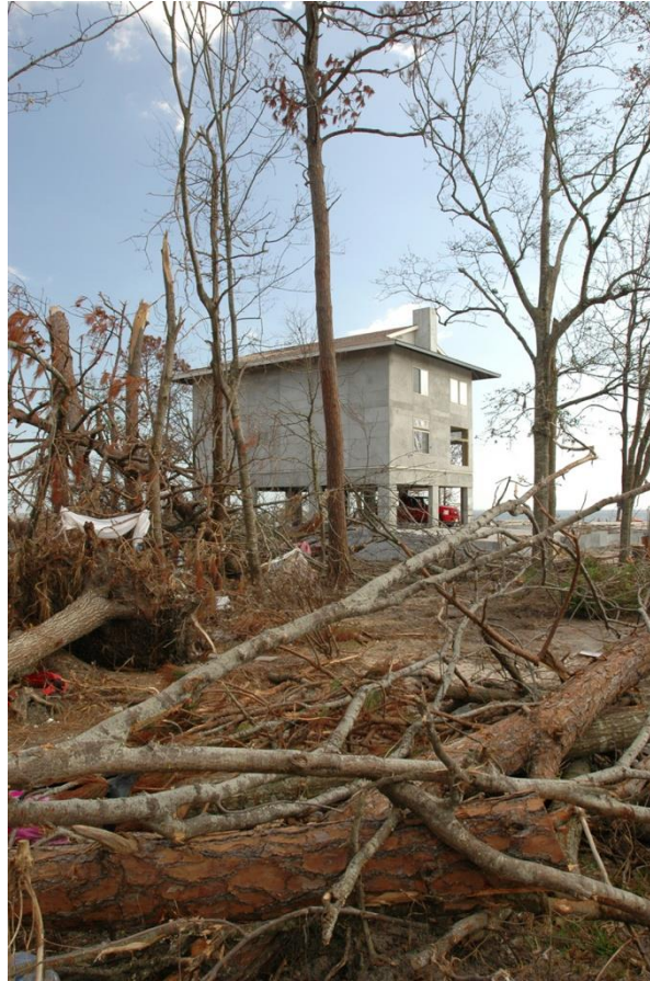
FIGURE 3.3: Pass Christian, Ms., Sep. 27, 2005—This Pass Christian (MS) home, which is constructed of steel reinforced concrete and closely follows hurricane-specific FEMA building standards, was the only house in its neighborhood to survive when Hurricane Katrina struck. Most other homes in the neighborhood were reduced to their foundations. Photo credit: John Fleck, FEMA, Sep. 27, 2005. Susie Shapira/FEMA.
