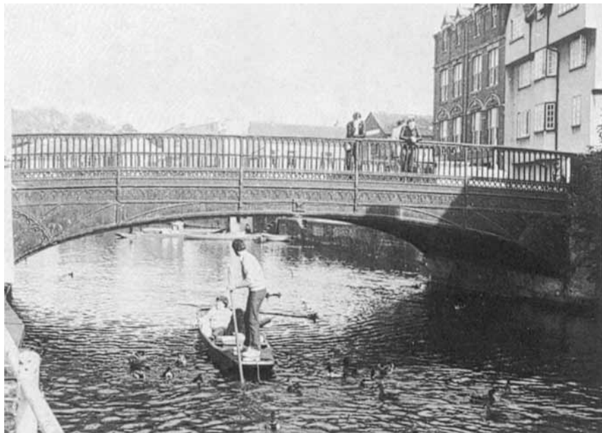
Figure 1.8 Magdalene Bridge built in 1823 on the site of the ancient Saxon bridge over the Cam. The present cast-iron arches carried, until recently, loads far in excess of those envisaged by the designers. Fortunately, the bridge has now undergone a well-earned restoration.
