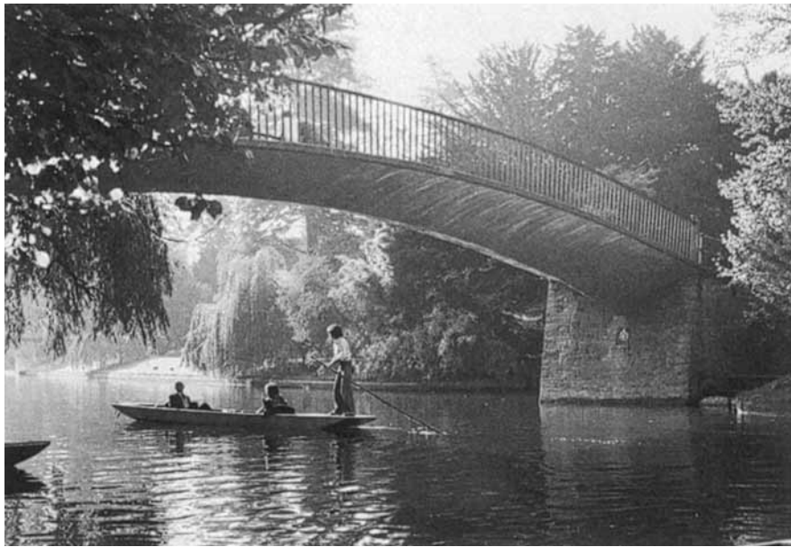
Figure 1.10 The reinforced concrete footbridge in Garret Hostel Lane. An inscription carved nearby reads: "This bridge was given in 1960 by the Trusted family members of Trinity Hall. It was designed by Timothy Guy MORGAN an undergraduate of Jesus College who died in that year."
