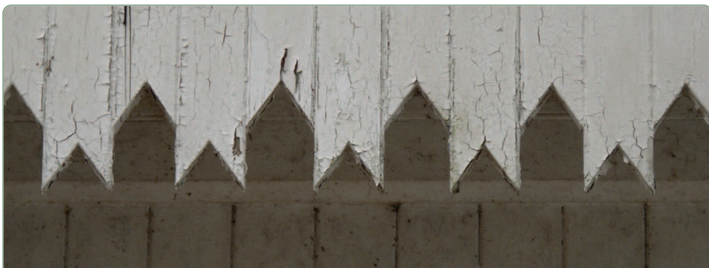
Traditional timber fascia detail, nineteenth-century railway station, Killin Pier
