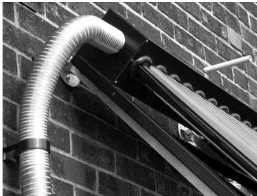
Well-insulated pipework and warm water recirculation is a new alternative to antifreeze in solar water heating installations (Reproduced with permission from Powertech Solar)
