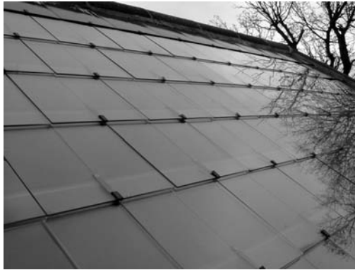
Toughened glass solar slates can replace an entire south facing roof (Reproduced with permission from Solex Energy Ltd)
