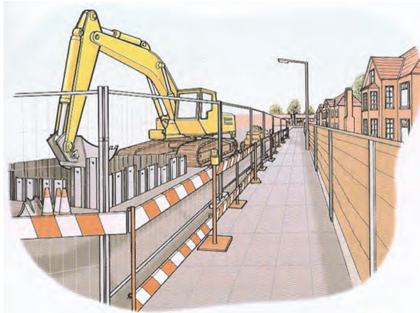
Figure 16.3 Barriers around excavation by footpath.
